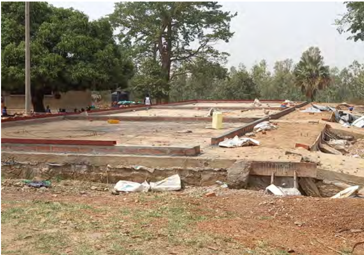
THE FOUNDATION FOR THE CLASSROOM BLOCKS BEING LAID
