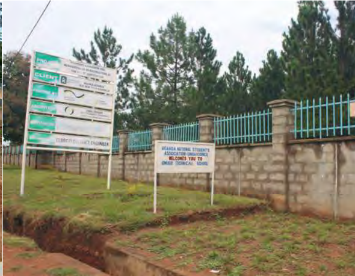
THE SCHOOL AFTER THE WALL CONSTRUCTION
