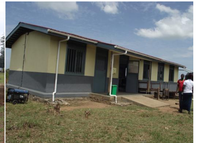
THE NEWLY CONSUTRUCTED INNOVATION CENTER
